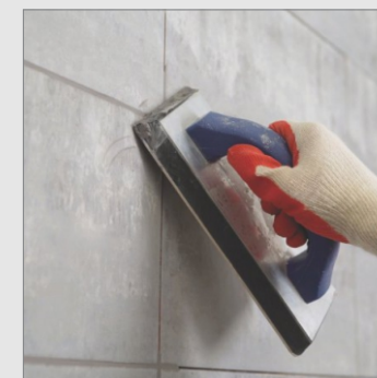
Joint Grouting
