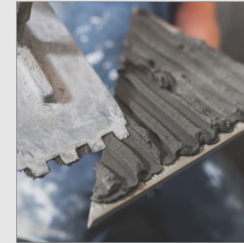
Cement Laying On Tile
