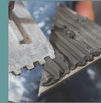
Cement Laying On Tile
